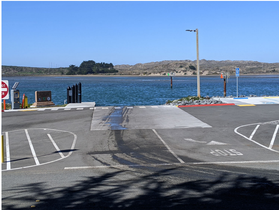
New concrete apron and path of travel between project elements
