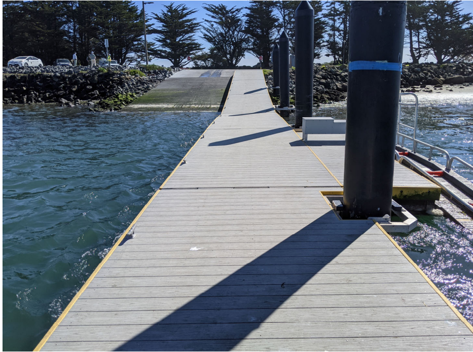
New pile guided boarding float with coated piles
