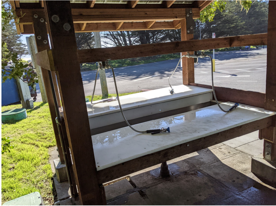
New fish cleaning station offers surfaces at two height levels to promote accessibility for all users
